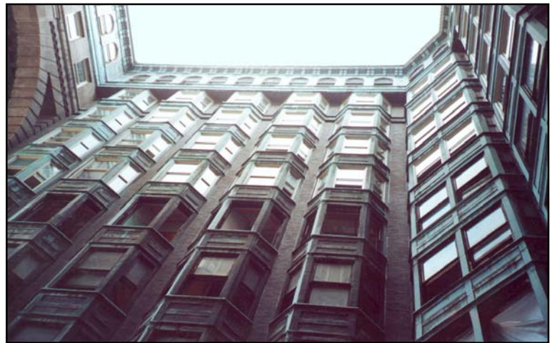
Restoration of the exterior copper required the crew to construct a 13-story scaffold around the U-shaped interior courtyard.
